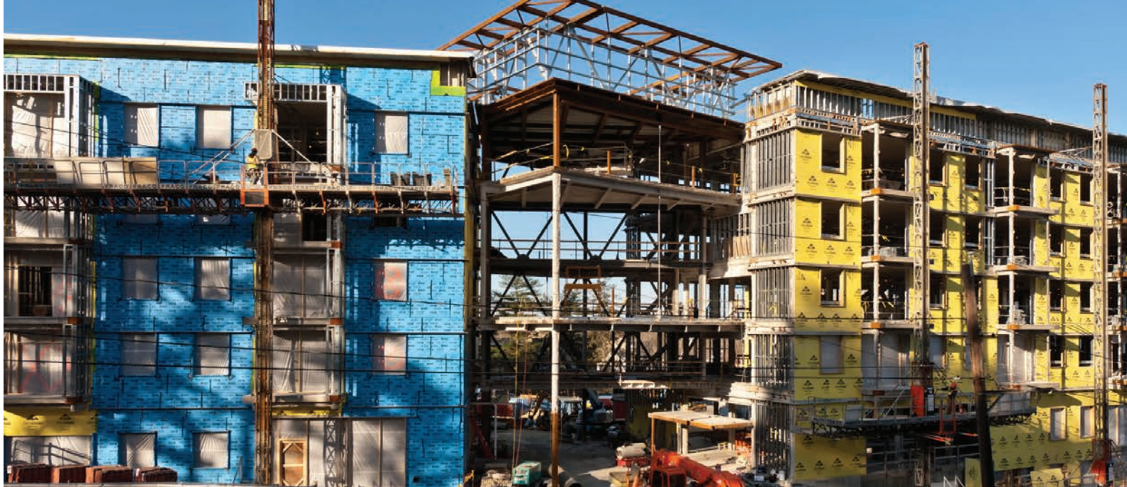
Image courtesy of Consigli Construction Co., Inc.
