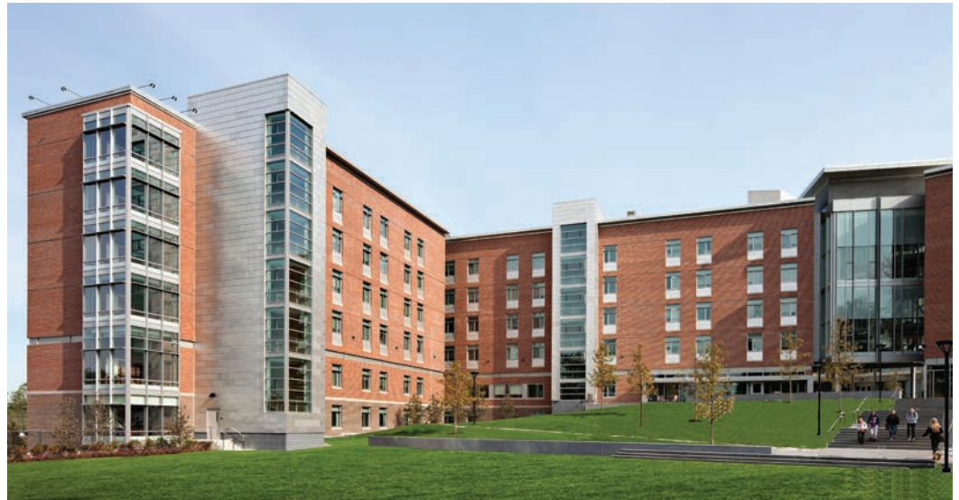
Image courtesy of Consigli Construction Co., Inc.
